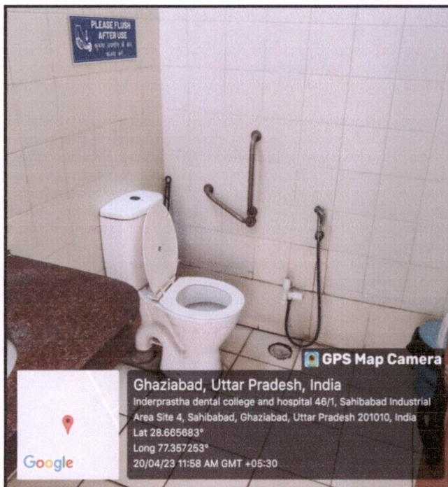
Disabled friendly washrooms
